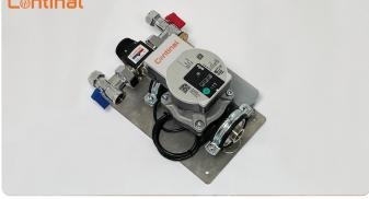
The HeatMax<sup>™</sup> small area mixer is designed to connect to new and existing heating systems with 15mm compression connections for the flow and return.
